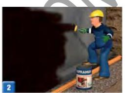
Then, two crosswise layers of **SOPRAKOTE** (0,6 L/m<sup>2</sup>/layer) are applyied. Alternatively, **SORPAMUR LATEX** is proposed.
