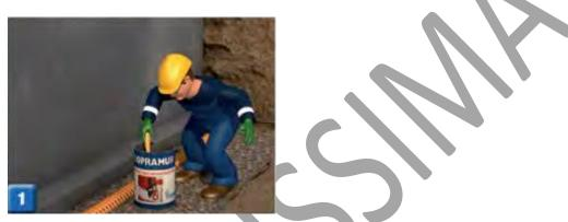
Application of a Primer layer elastomeric bituminous aqueous base lacquer **SOPRAKOTE**, diluted with 50% water. (0,3 L/m<sup>2</sup>). Alternatively, **SOPRAMUR LATEX** is proposed.
